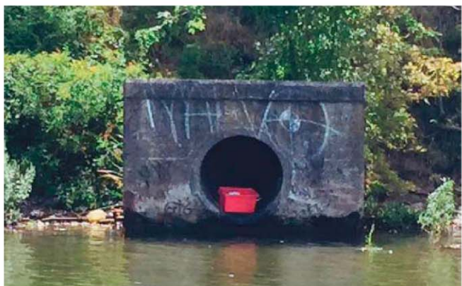
Combined sewer outfall
