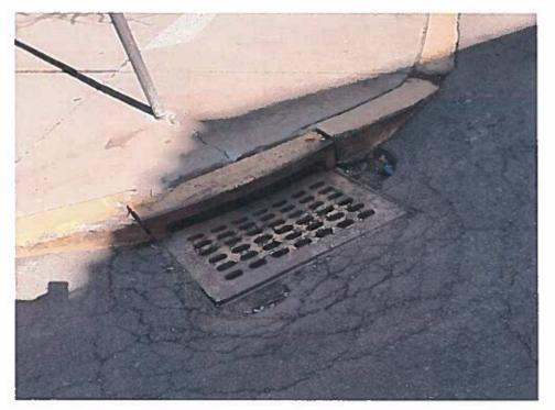
DESCRIPTION Collapsed catch basin RECOMMENDATION Repair collapsed catch basin
