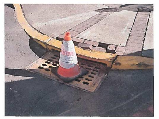
DESCRIPTION Collapsed catch basin RECOMMENDATION Repair collapsed catch basin APPROVED-----
