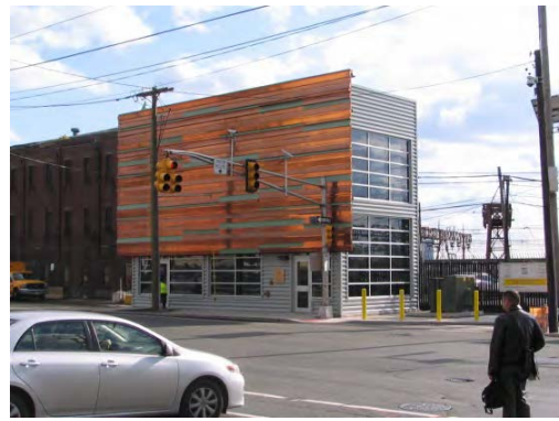
Completed H1 WWPS Electrical and Controls Building
