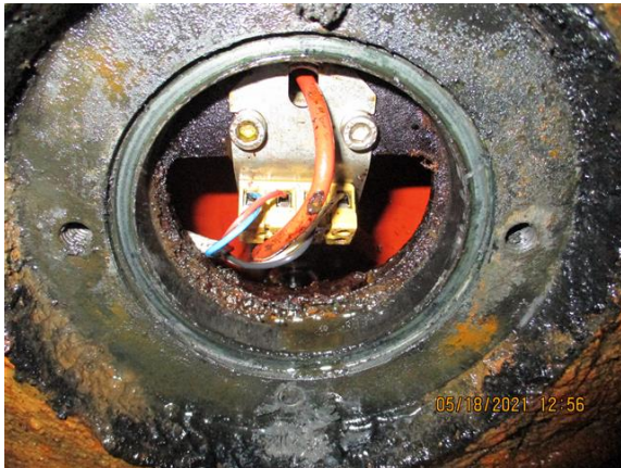
9- Seal Fail Inspection
