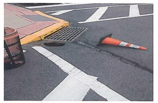
DESCRIPTION Collapsed catch basin RECOMMENDATION Repair collapsed catch basin
