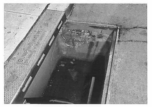
DESCRIPTION **Collapsed catch basin** RECOMMENDATION Repair collapsed catch basin
