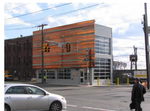
Completed H1 WWPS Electrical and Controls Building
