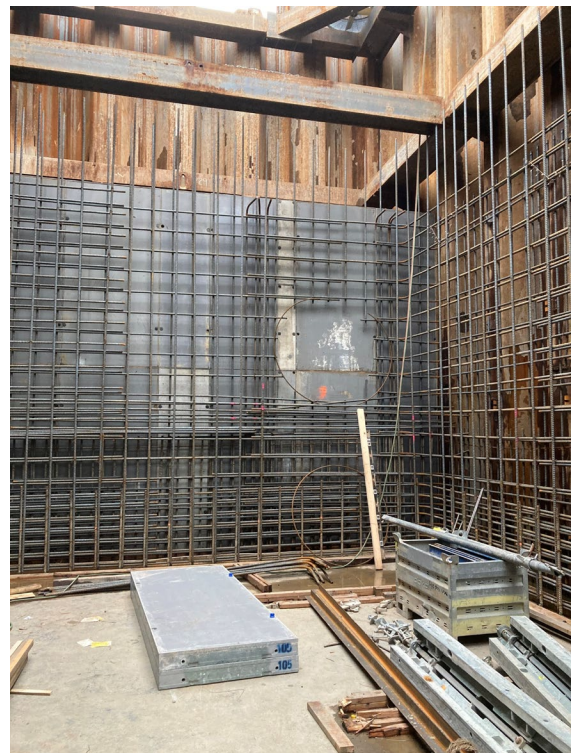
Pump Station being installed in phase 1.
