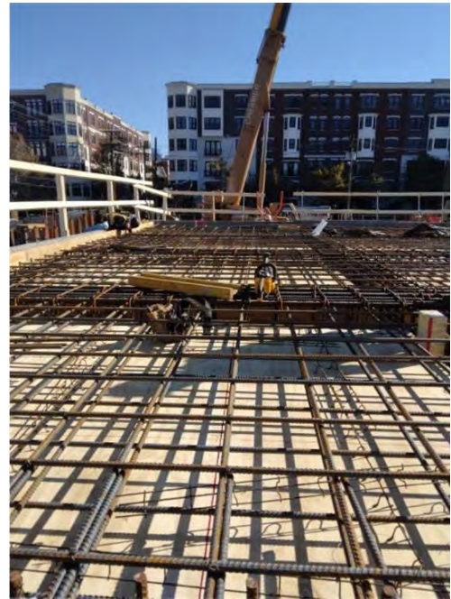
Construction of New Control Building in Phase 1
