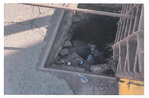
DESCRIPTION Collapsed catch basin RECOMMENDATION Repair collapsed catch basin
