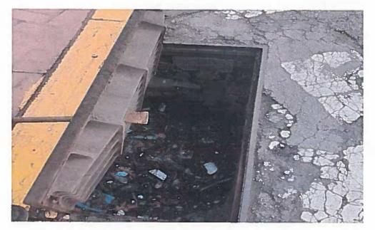
DESCRIPTION Collapsed catch basin RECOMMENDATION Repair collapsed catch basin
