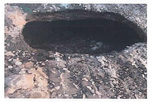
DESCRIPTION Collapsed catch basin lateral RECOMMENDATION Repair collapsed lateral
