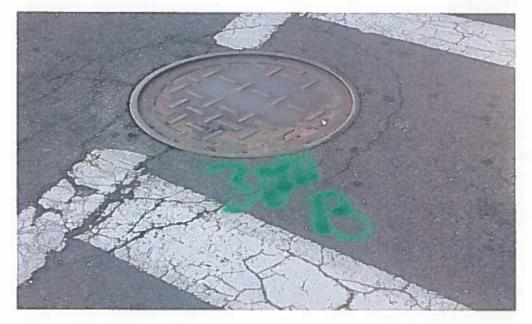
DESCRIPTION Severely worn manhole casting RECOMMENDATION Replace manhole casting
