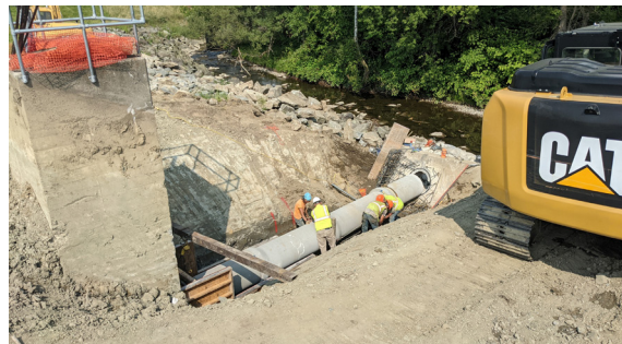
NYS OGS Levee Outfall Conduit Replacement, Endicott, NY.
