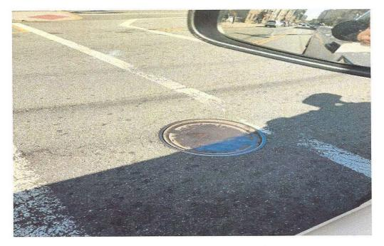
DESCRIPTION Severely worn manhole casting RECOMMENDATION Replace manhole casting
