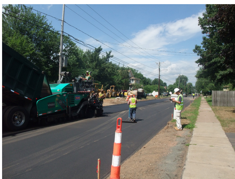
Goodwin Street paving operations for East Hartford Roads CEI
