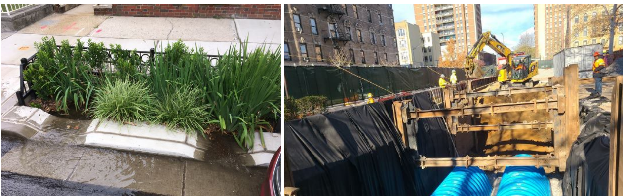
Left: A completed bioswale collecting water from a city street
