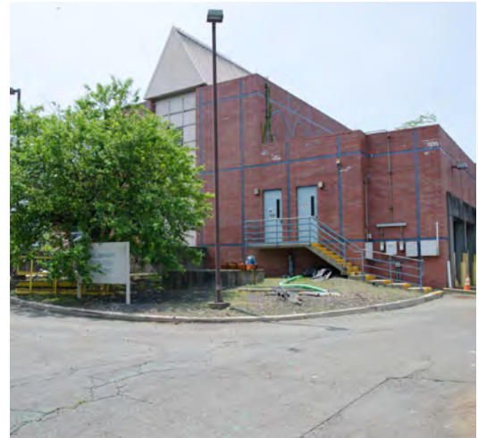
Potential site of the Grand Street Pumping Station at the Adam Street WWTTP
