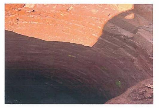
DESCRIPTION Collapsed manhole RECOMMENDATION Repair collapsed manhole
