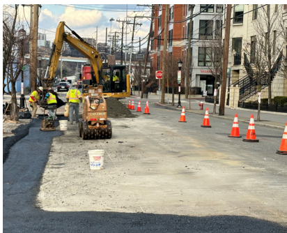
Temporary Asphalt Paving Madison Street Area Infrastructure Improvement Phase 1
