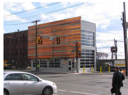
Completed H1 WWPS Electrical and Controls Building
