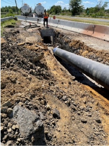
Horizontal directional drilling in progress.
