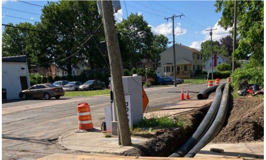
Northern Interceptor Project: Routing bypass force main under Connecticut Boulevard.
